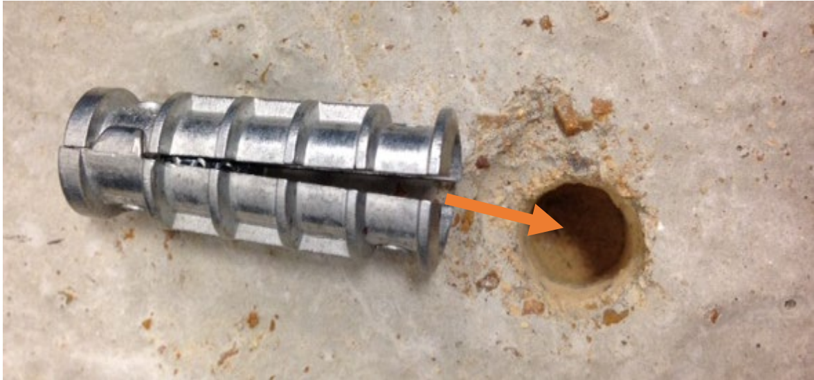
Figure 29: Anchor with expanded end pointing to hole
