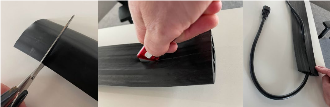
Figure 31: Cable protector: left (cut protector length), middle (cut to slice open protector cavity), right (slide cable into protector cavity)
