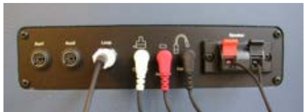
Figure 3: Cable placement in TBS25
